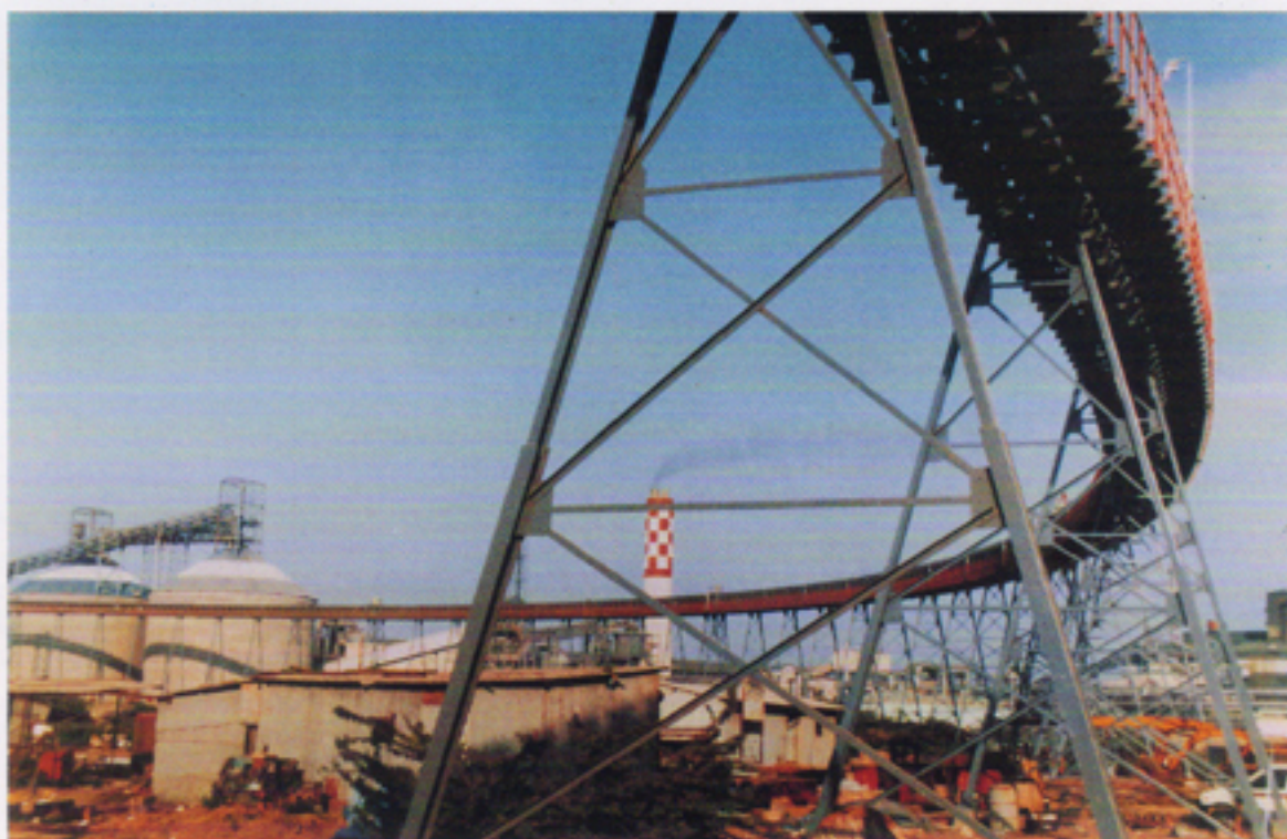
Fig.1: 3.2 km long pipe conveyor at Birla Copper
